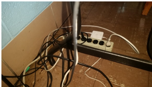
Insufficient Power Receptacles
