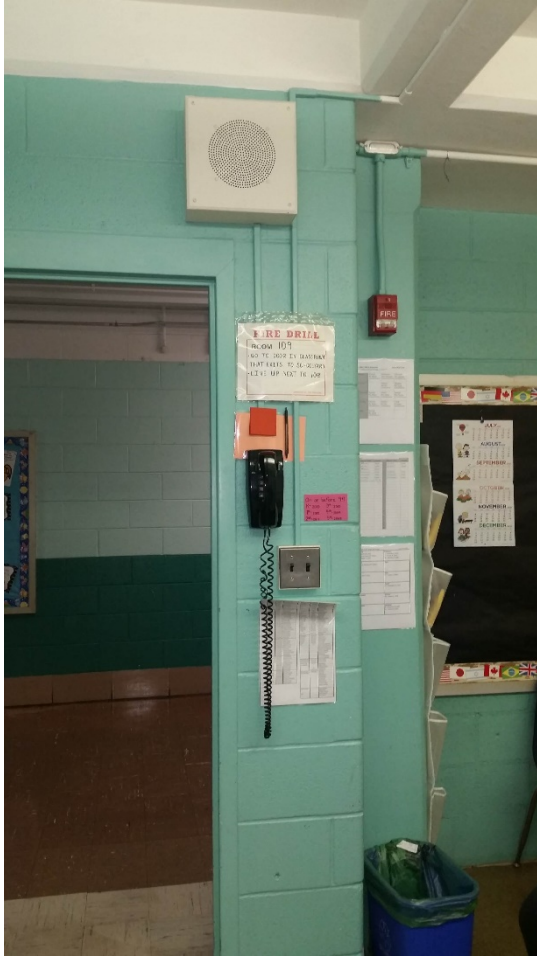
Typical Phone, PA speaker and Bell System
