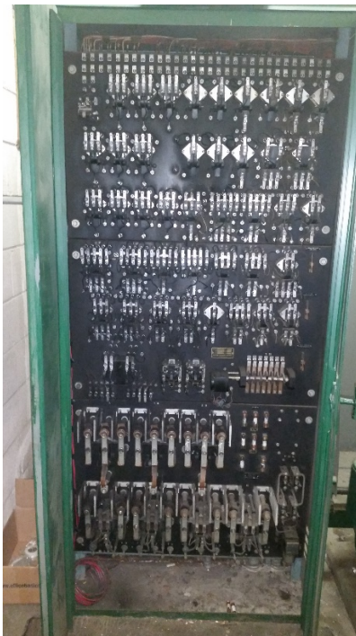
Elevator Control Panel
