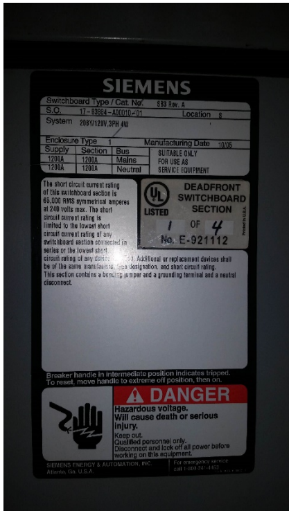
Main Switchboard Nameplate
