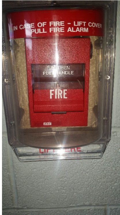
Typical Fire Alarm Pull Station
