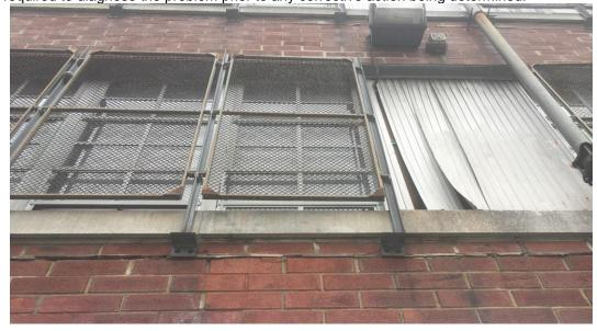
Existing exterior doors and frames are in fair to poor condition. Deterioration of frames and doors at several locations is extreme. There are eighteen pairs of double doors and four single leaf door serving the first floor. Two separate storefront systems with double doors will be replaced in their entirety. Existing roof access door to remain.
