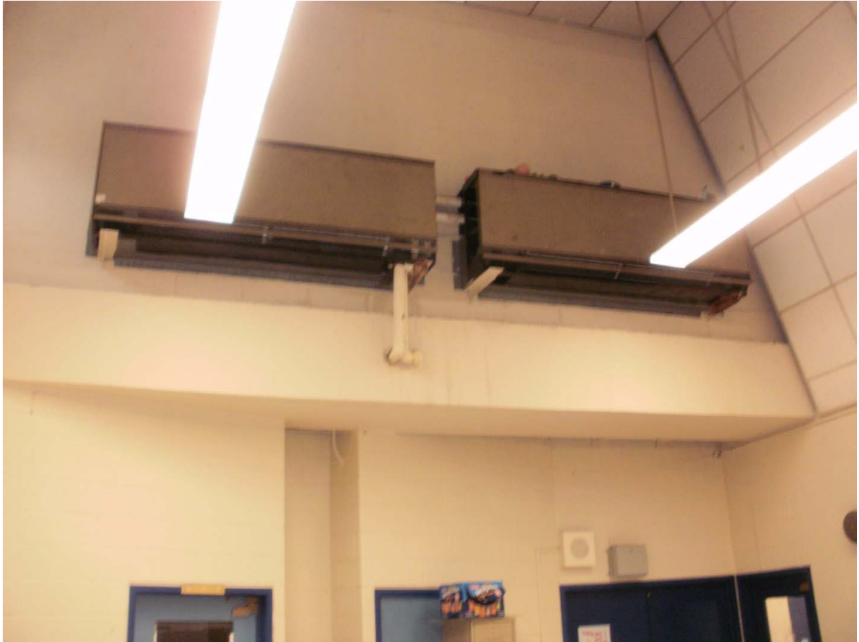
Photo No. 5 – Atypical Classroom Unit Ventilator Coil, Filter and Fan Assembly.
