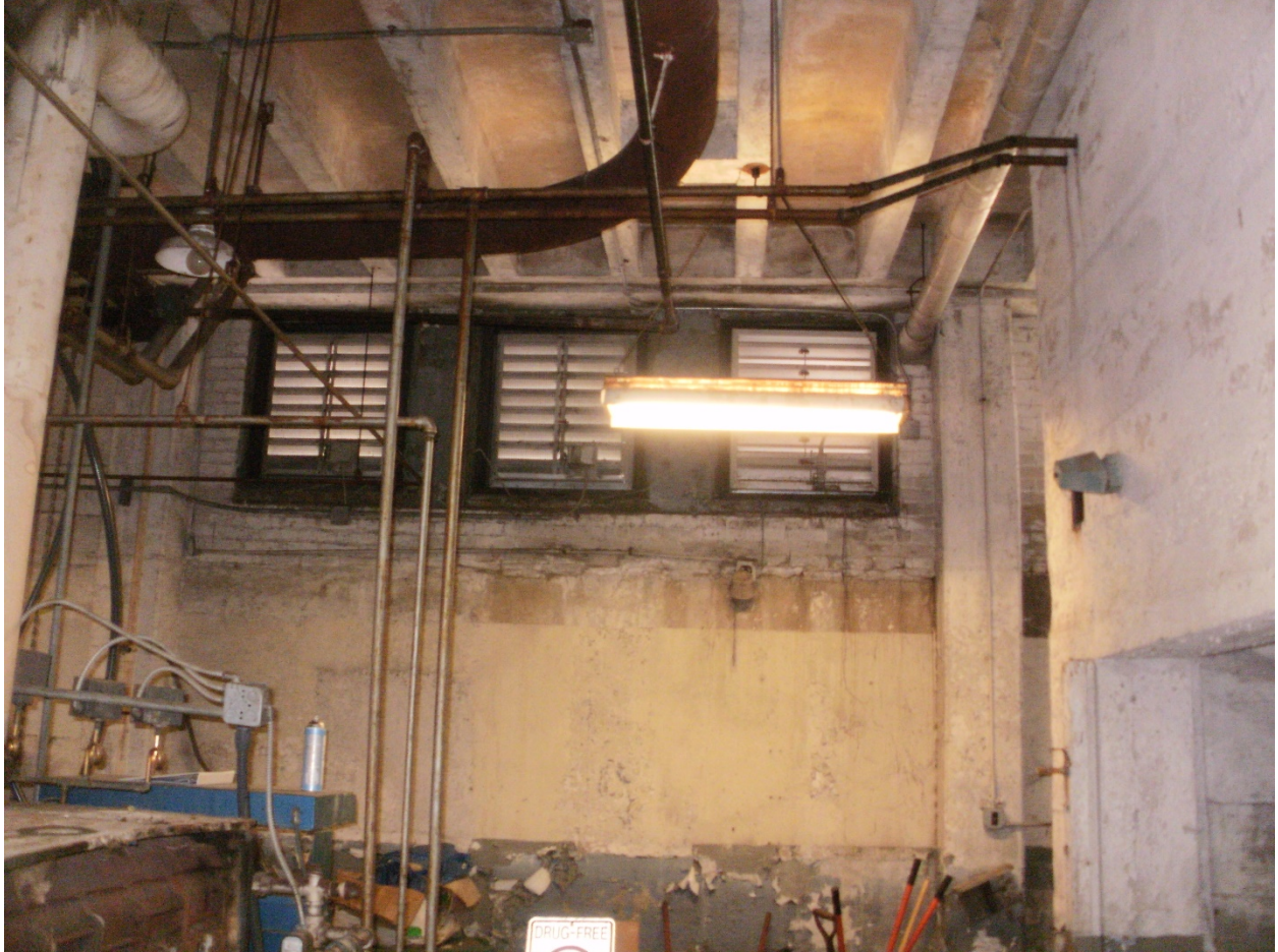
Photo No. 7 - Boiler Room Combustion Air Louvers
