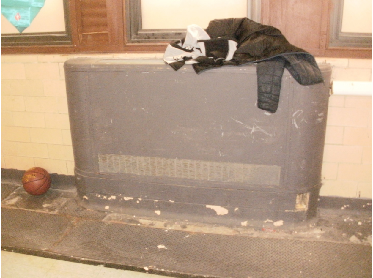
Photo No. 9 – A typical surface mounted low pressure steam radiator located in the gym
