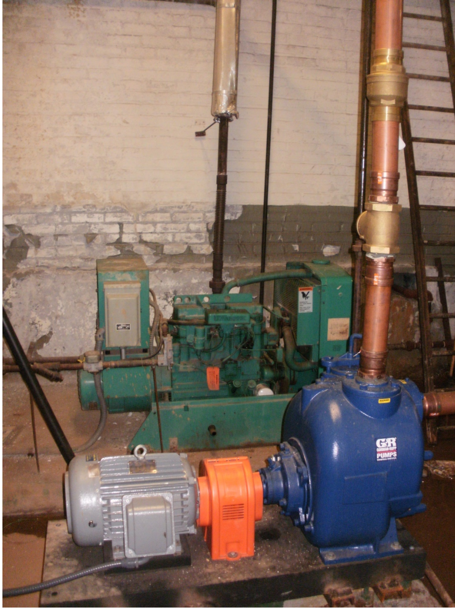
Photo No. 5 – Supply Pump and Emergency Generator
