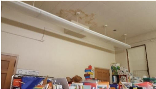
ACT Ceiling Damage @ K Coatroom 100A
