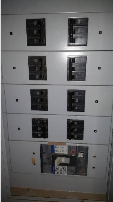
Main Distribution Panel
