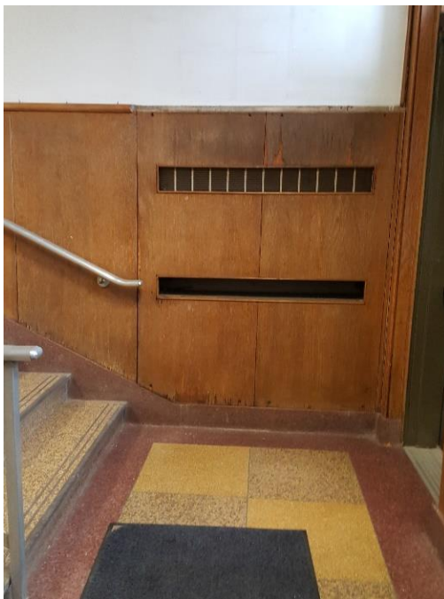
Wood panel wainscot @ Main Entrance
