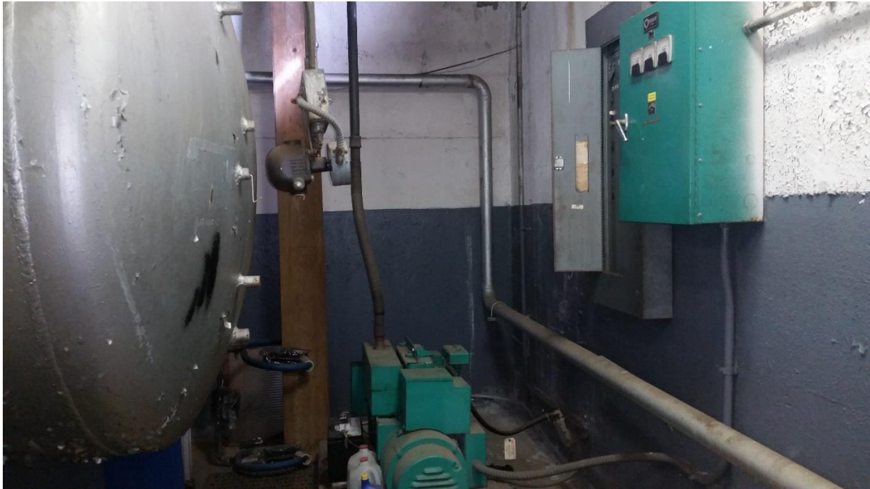
Existing Generator, Emergency Panel and ATS
