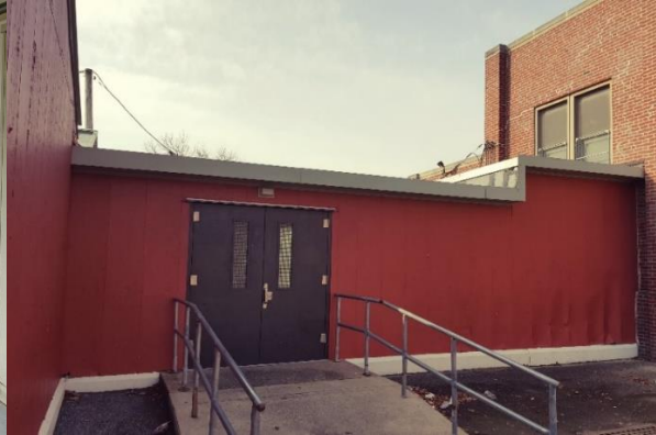
Annex Connector Corridor Exterior
