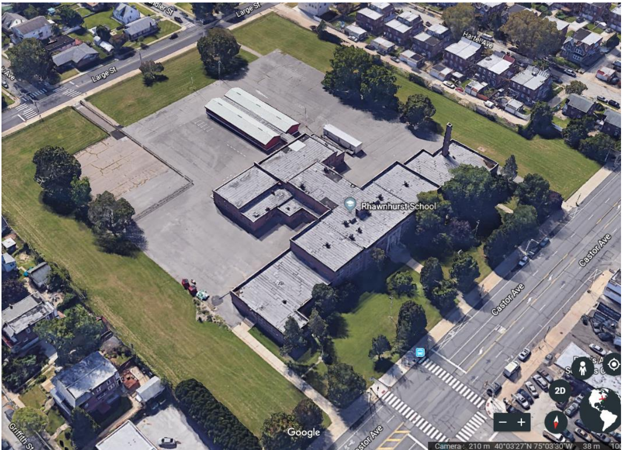
Aerial View of Site
