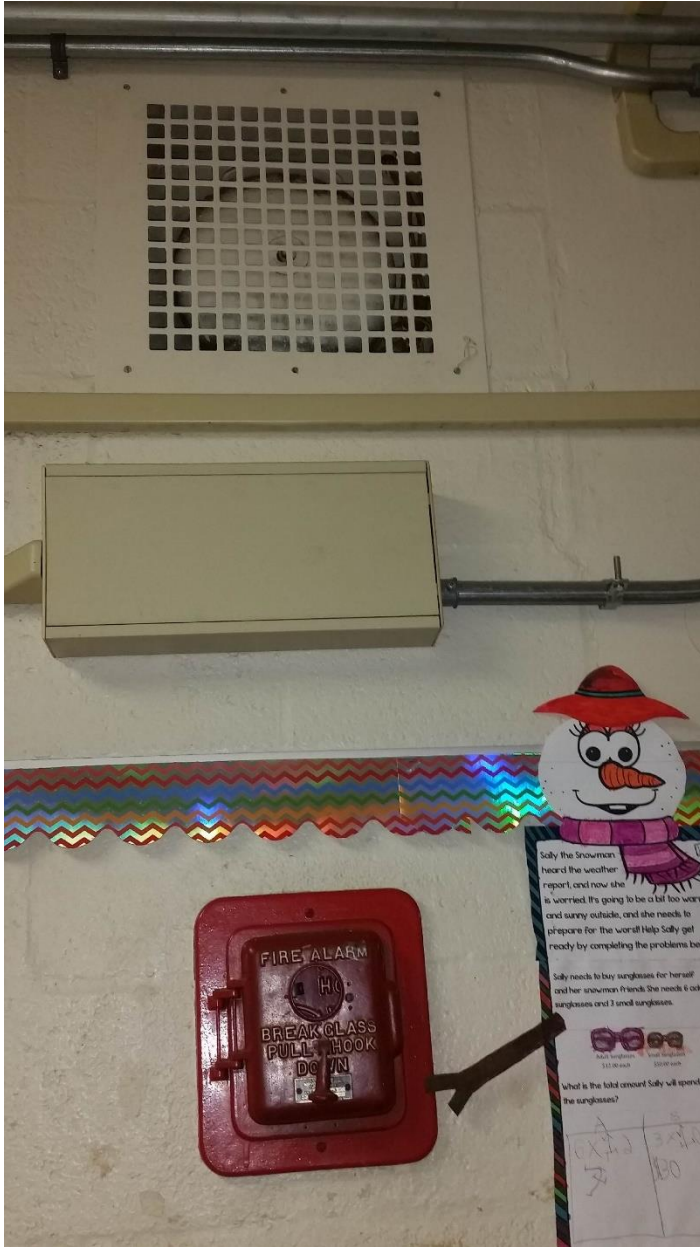
Typical Fire Alarm Gong and Typical Fire Alarm Pull Station
