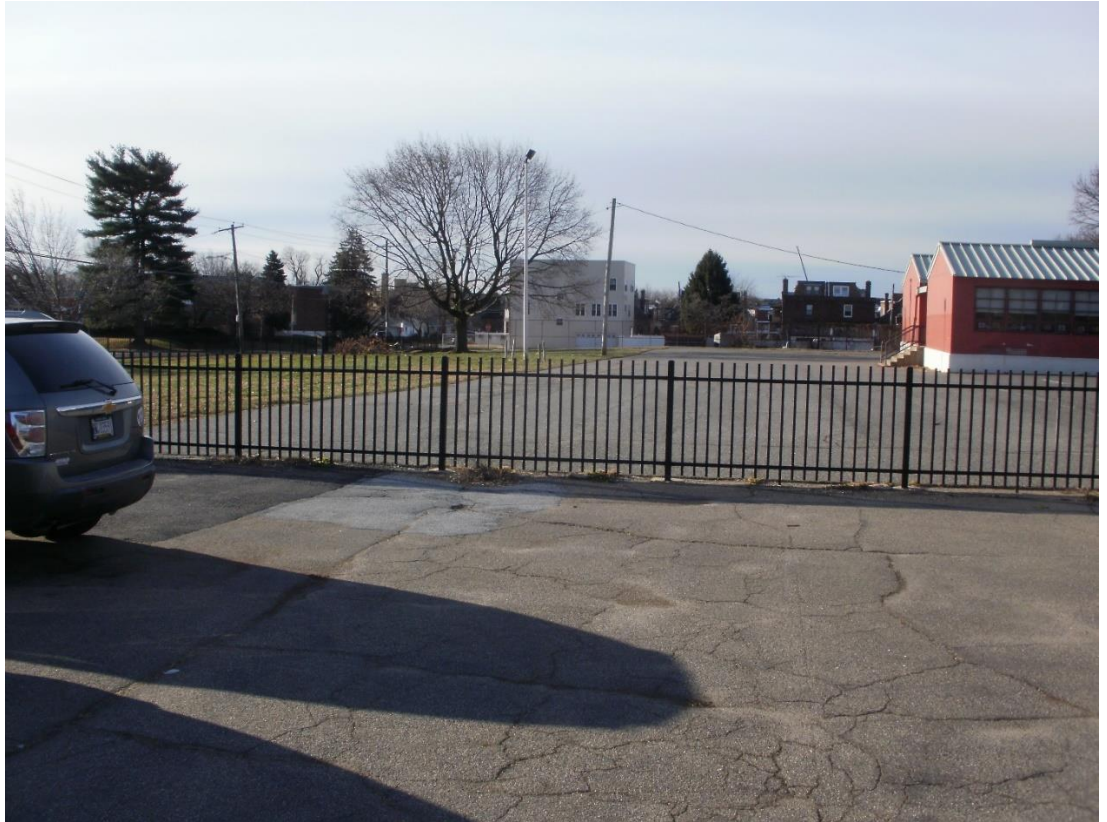
View of Pavement @ Parking Lot
