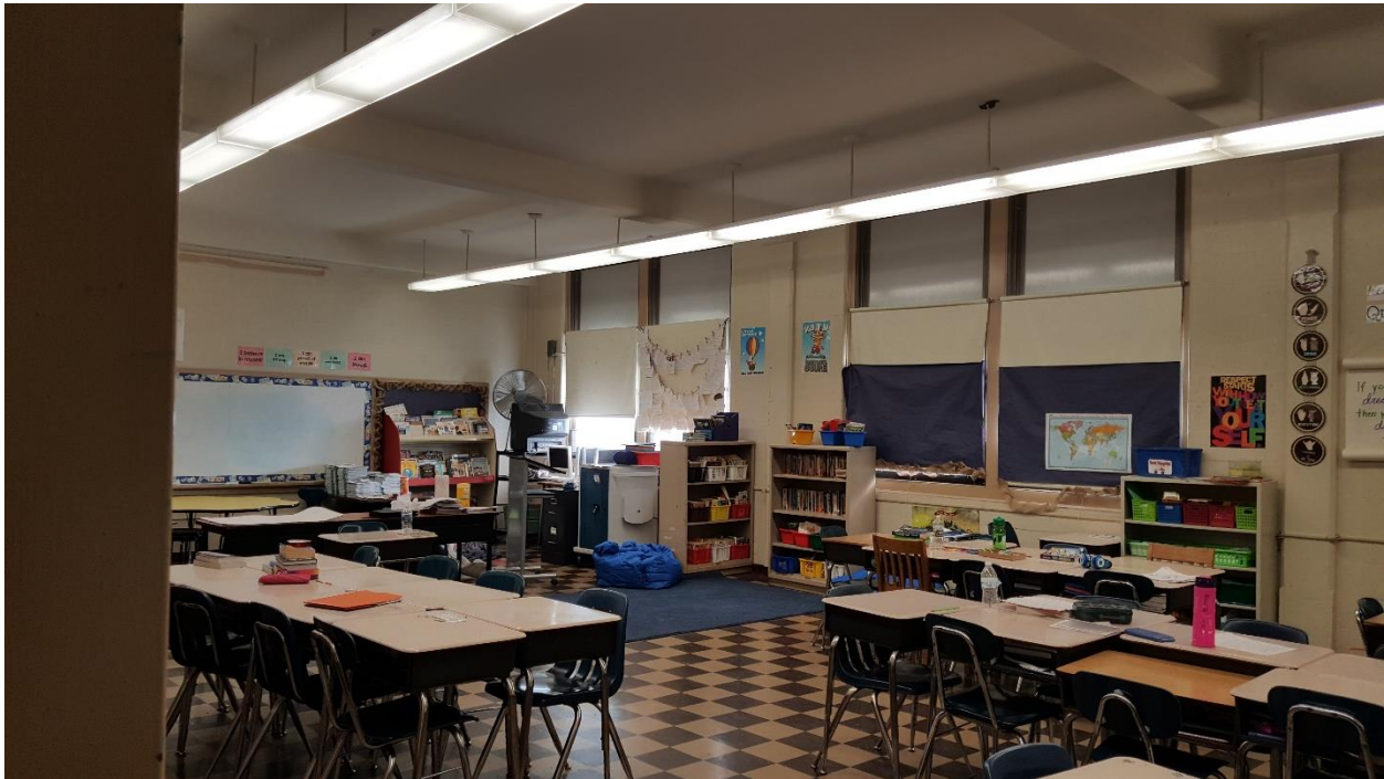
Typical Classroom Lighting @ Main Building
