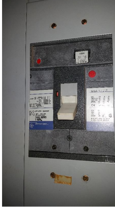
Main Distribution Panel Overcurrent Protection 600A
