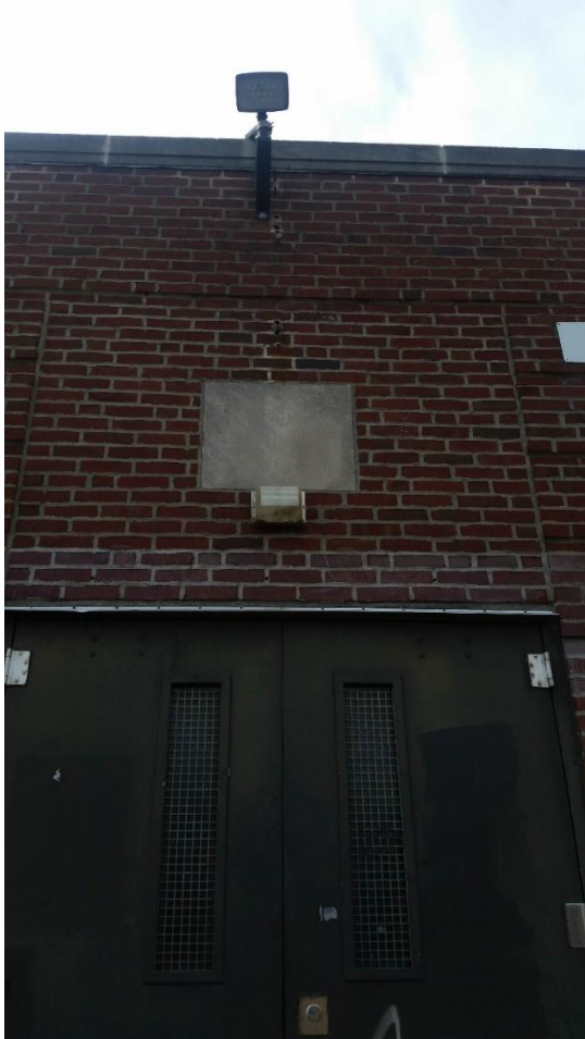
Typical Exterior Lighting
