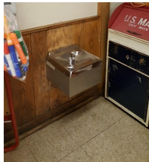
Wood panel wainscot at drinking fountain
