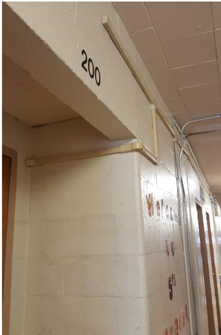
CMU block walls @ Main Corridor
