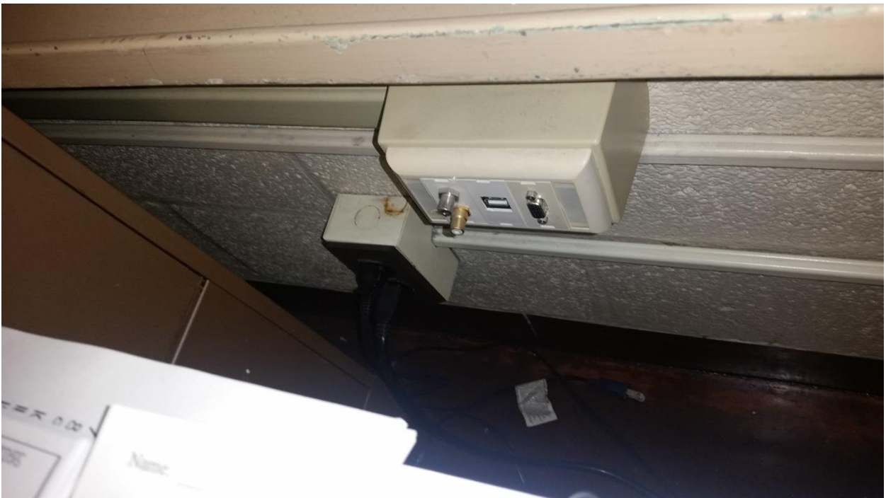
Insufficient Power Receptacles
