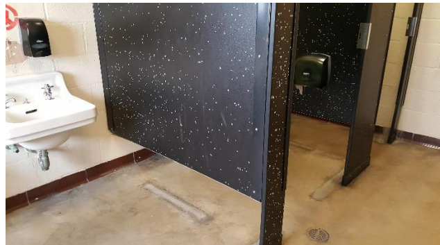
Concrete floor in bathrooms
