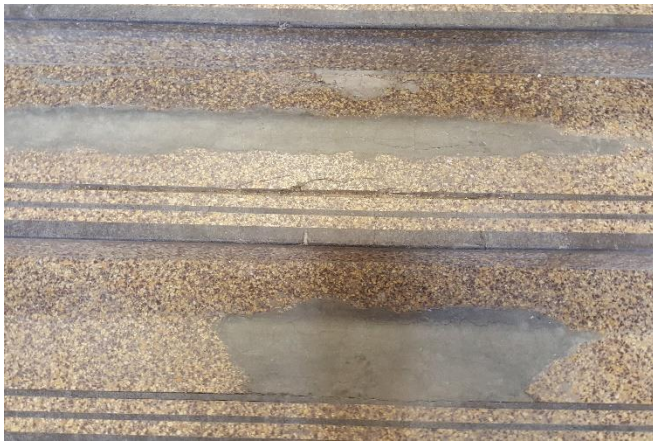
Concrete floor in stairway
