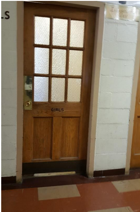
Typical bathroom doors and hardware to be replaced
