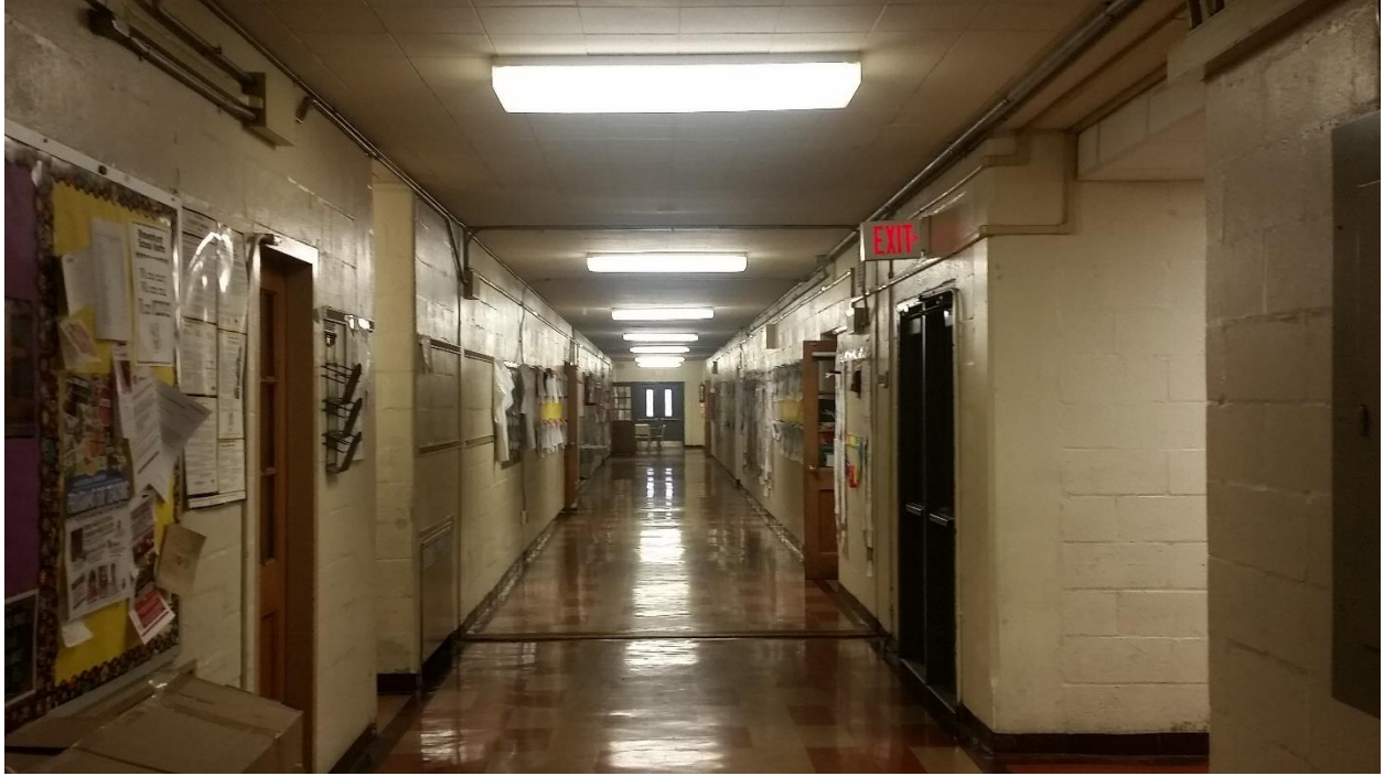
Typical Corridor Lighting @ Main Building
