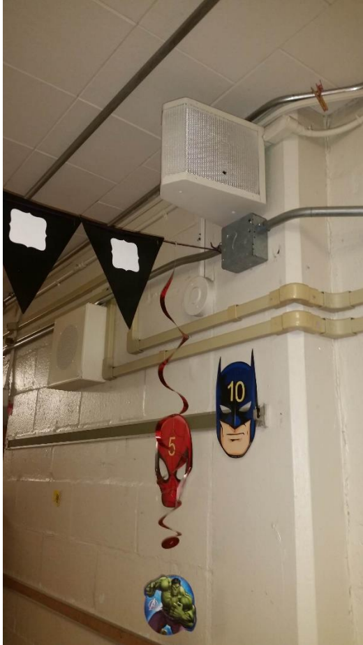
Typical Decommissioned PA Stainless Steel Speaker Typical Square PA Speaker Currently In Use
