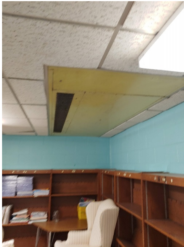
Photo No. 12 – A typical ceiling mounted unit ventilator
