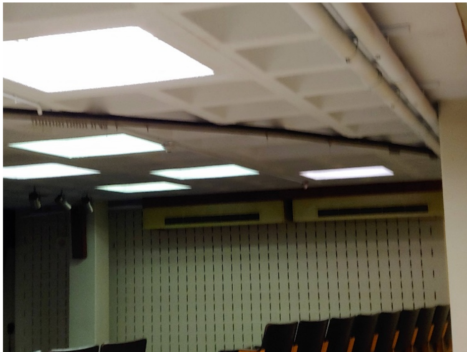
Photo No. 14 – Two surface mounted unit ventilators located in Cafetorium
