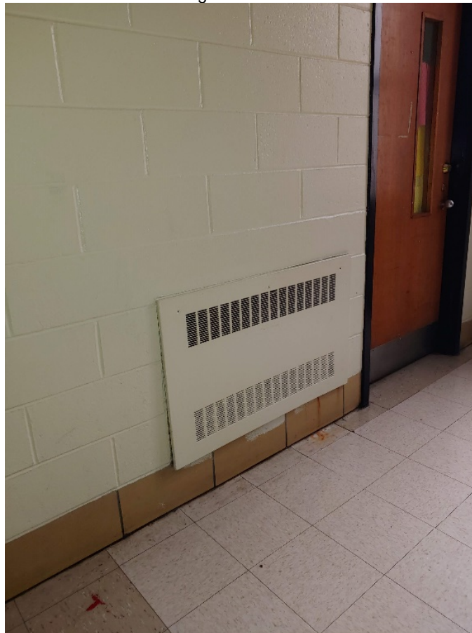
Photo No. 16 – Existing recessed wall mounted radiator
