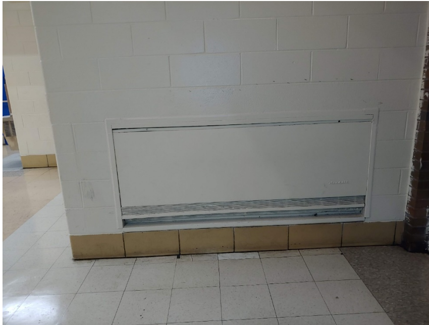
Photo No. 16 – Existing recessed wall mounted radiator
