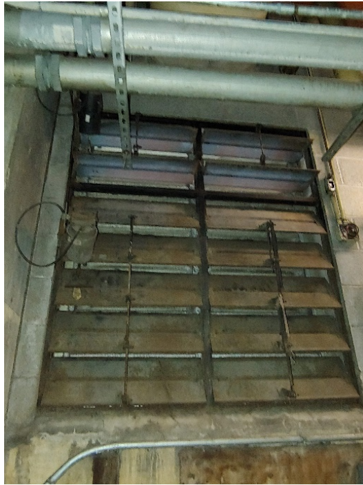
Photo No. 5 – Boiler Room Combustion Air Louvers
