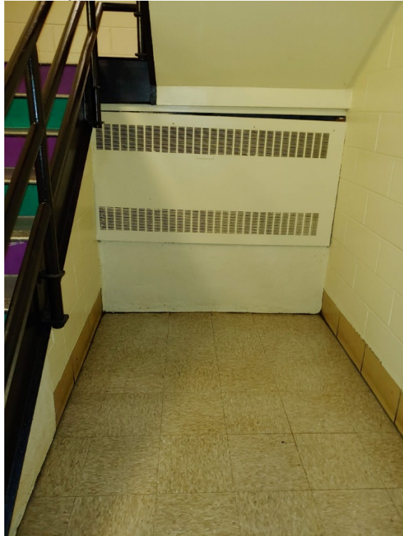
Photo No. 10 – A typical recessed radiator located in the corridor area.
