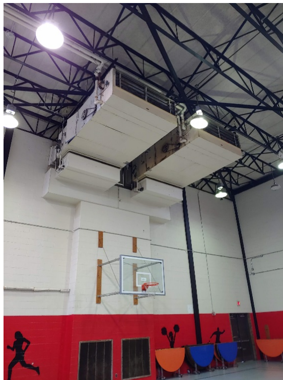
Photo No. 8 – H & V Units 1 & 2 located in the gym ceiling area.
