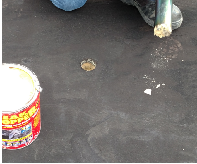
3. Roof core sample.
