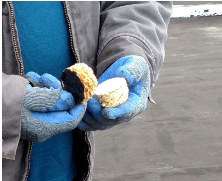
4. Detail, roof core sample.
