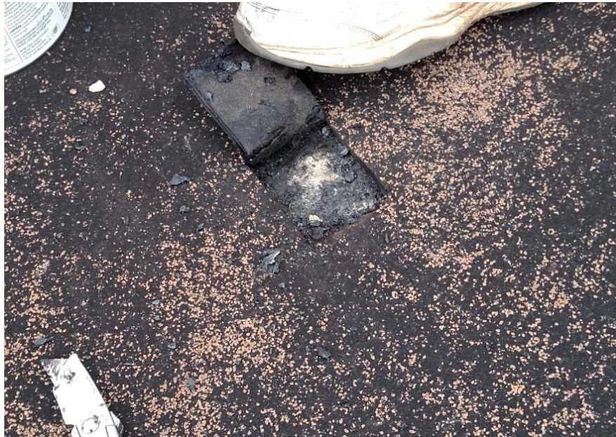
Roof membrane adhered to concrete deck showing degraded granular coating
