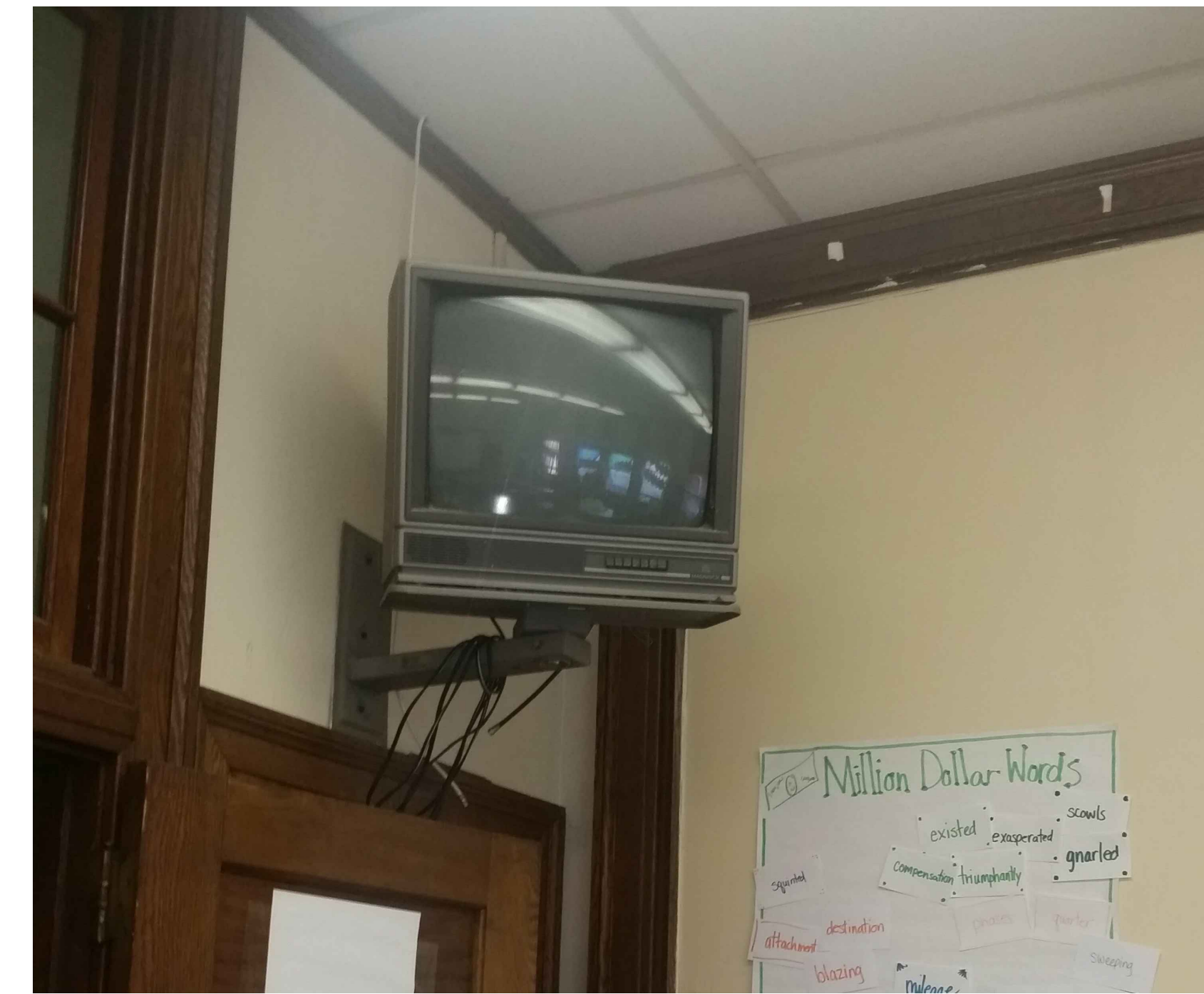
EXISTING TV TYPE AND ASSOCIATED MOUNTING BRACKETS AND HARDWARE TO BE REMOVED
