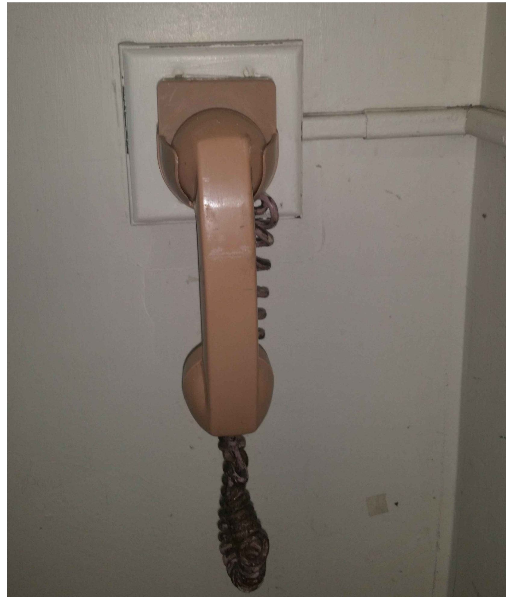
EXISTING WALL PHONE TYPE TO BE REMOVED
