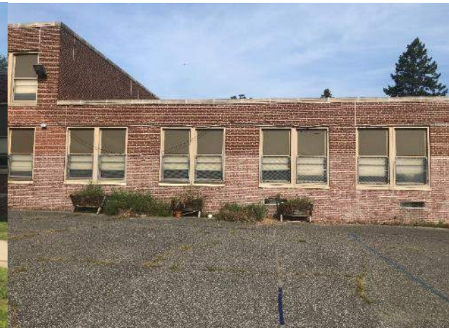
C CLASSROOM WING FACING HARD SURFACE PLAY AREA AND LARGE STREET
