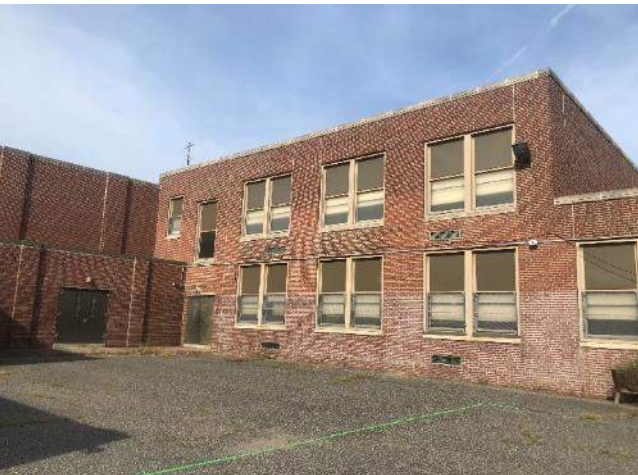
D TWO STORY CLASSROOM WING FACING HARD SURFACE PLAY AREA AND LARGE STREET
