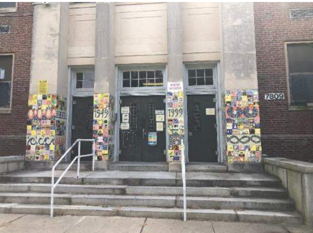
A MAIN ENTRANCE FACING CASTOR AVENUE
