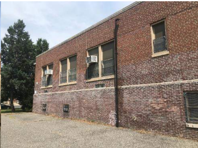
E CLASSROOM WING FACING HARTEL AVENUE
