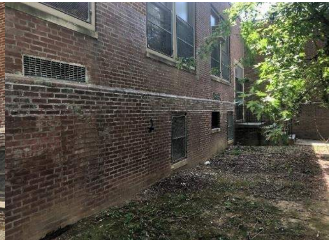
F SIDE ENTRANCE TO CLASSROOM WING FACING CASTOR AVENUE
