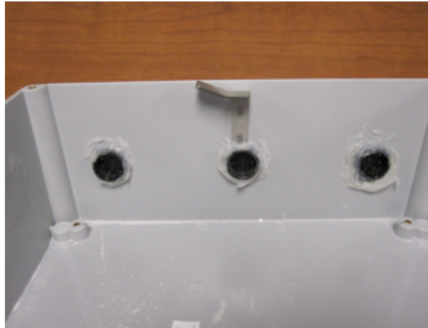
Figure 4. Interior view of vent plugs.
