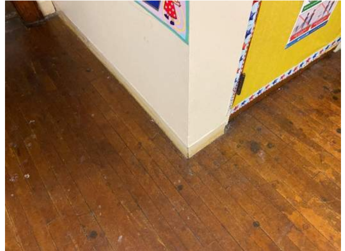
Photograph 2: HID 03. Covebase Mastic (non-ACM)
