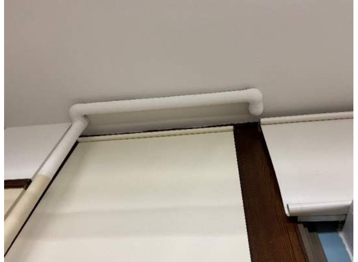
Photograph 6: HID 9. Pipe Fitting Insulation ( Previously Confirmed ACM ) and HID 10. Pipe Insulation 2-6 Inch ( Previously Confirmed ACM )
