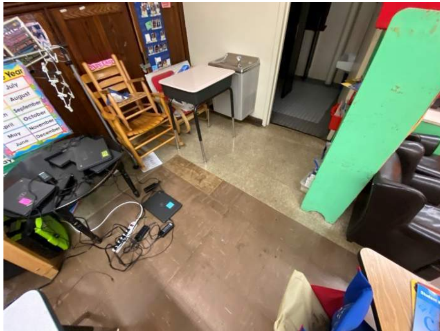
Photograph 7: HID 7. 12"x12" Tan Floor Tile and Mastic (NAD/NAD) and HID 14. Floor Tile VAT 9"x9" Brown ( Previously Confirmed ACM )
