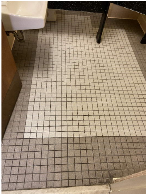
Photograph 3: HID 04. Ceramic Tile Wet Bed (NAD)
