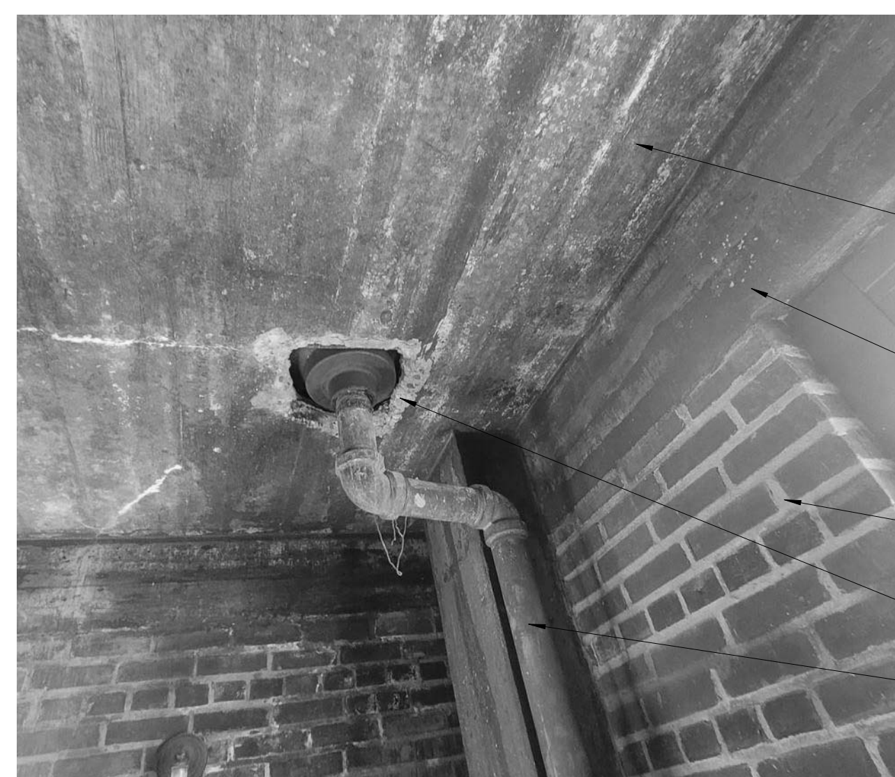
PHOTO B - SPALLED CONCRETE CEILING SLAB
