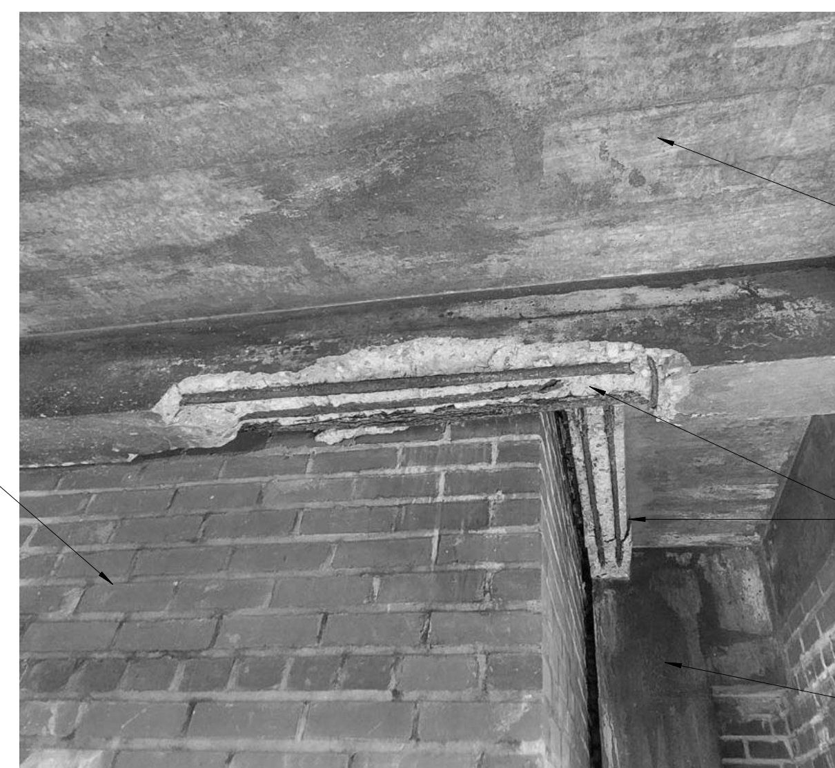
PHOTO A - SPALLED BEAMS WITH EXPOSED REBARS
