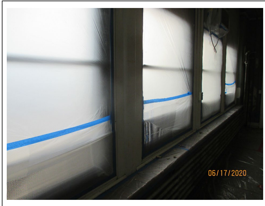
Photograph 9 – Classroom windows sealed for stabilization
