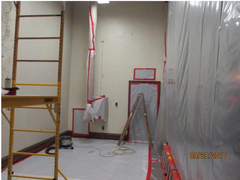
Photo 16 – Interior Containment: Cover Floors, Curtains, and Openings on Stage.
