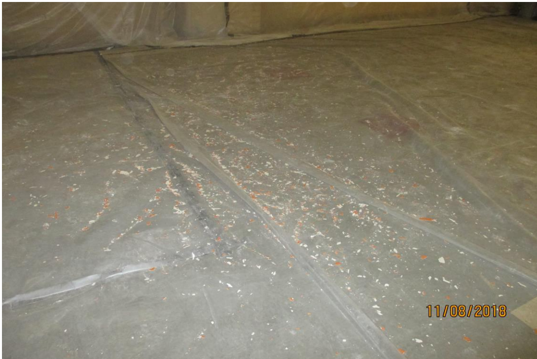
Photo 14 – Removed Flaking Paint Chips in Gymnasium Containment Area.
