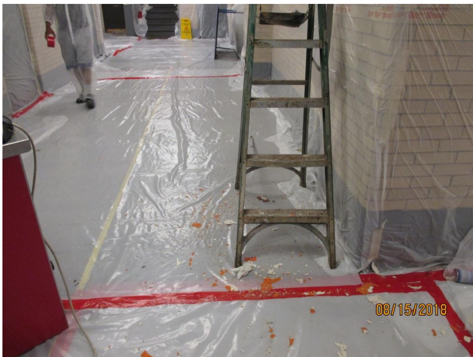
Photo 7 – Interior Containment/Scraping: Cover Floors and Walls (in Basement Hallway).
