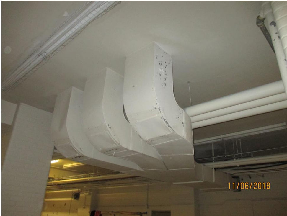
Photo 11 – Flaking Paint prior to Scraping in Gymnasium Containment Area.
