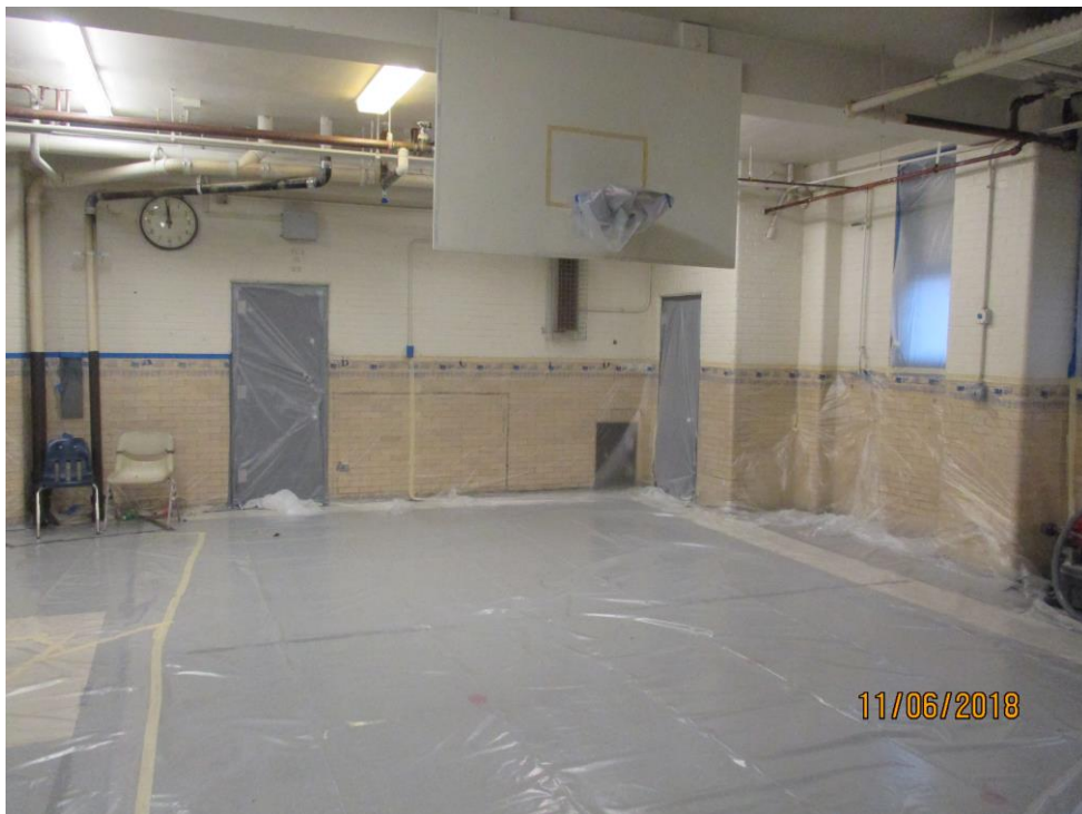
Photo 10 – Interior Containment: Cover Floors, Objects, and Walls (in Gymnasium).
