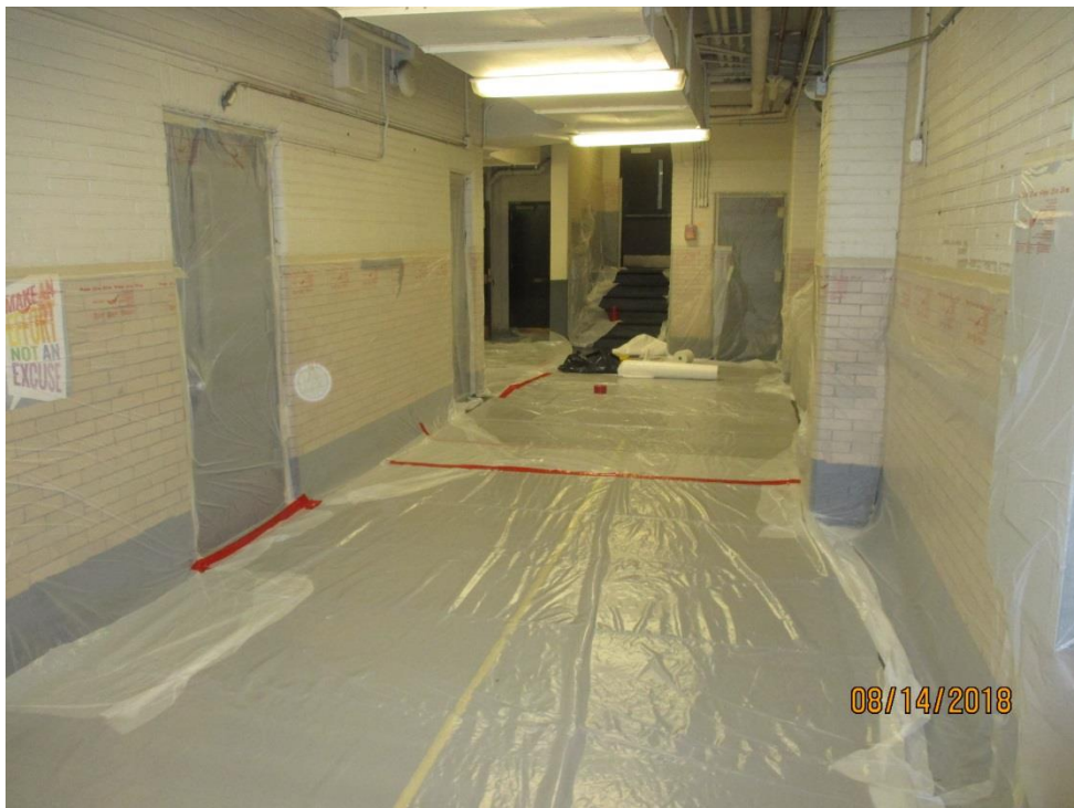
Photo 6 – Interior Containment: Cover Floors and Walls (in Basement Hallway).
