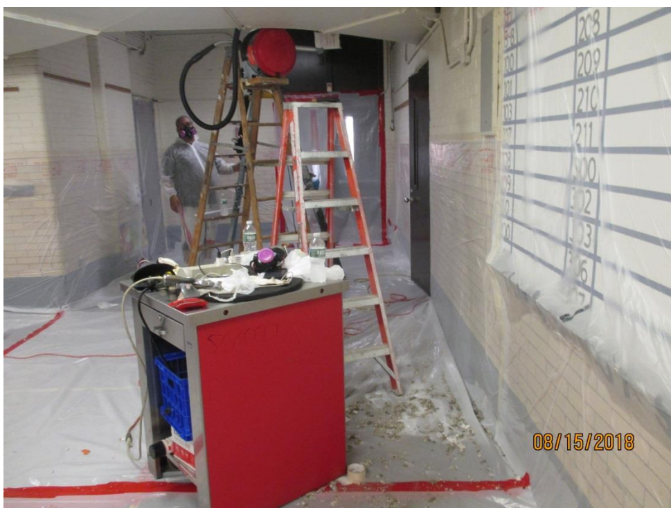
Photo 8 – Scraping/Removing Flaking Paint in Basement Hallway Containment Area.
