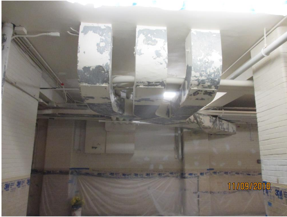
Photo 13 – Scraping/Removing Flaking Paint in Gymnasium Containment Area.
