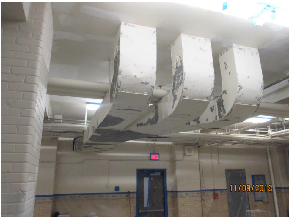
Photo 12 – Scraping/Removing Flaking Paint in Gymnasium Containment Area.
