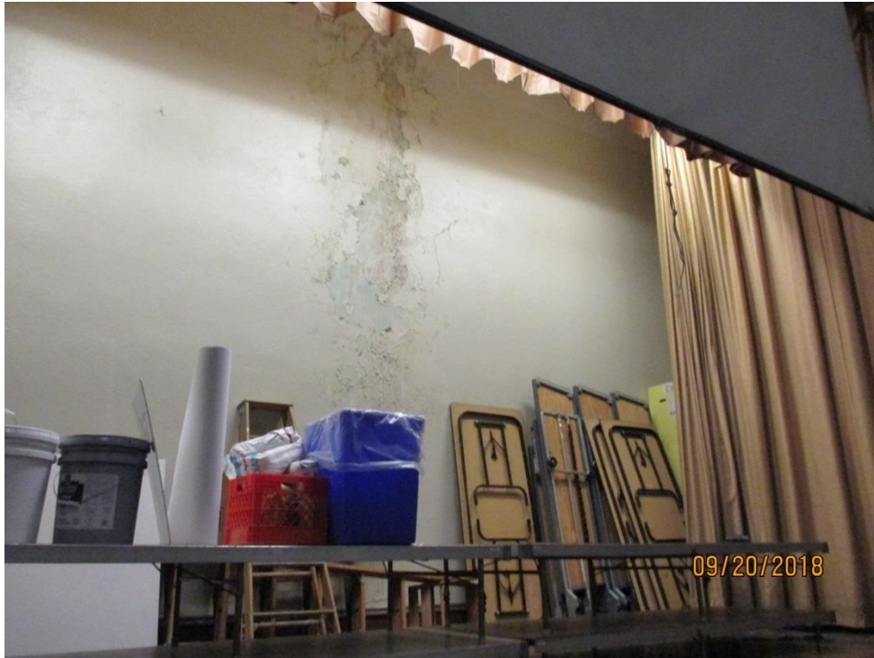
Photo 17 – Stage Wall Damage Prior to Prepping and Scraping.
