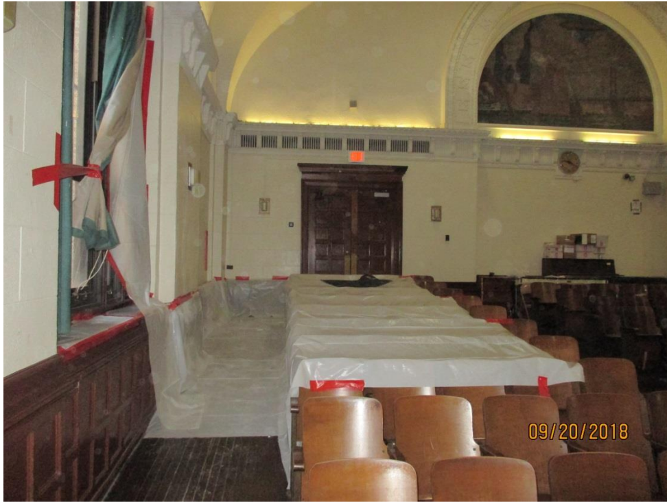
Photo 15 – Interior Containment: Cover Floors and Chairs in Section of Auditorium.
