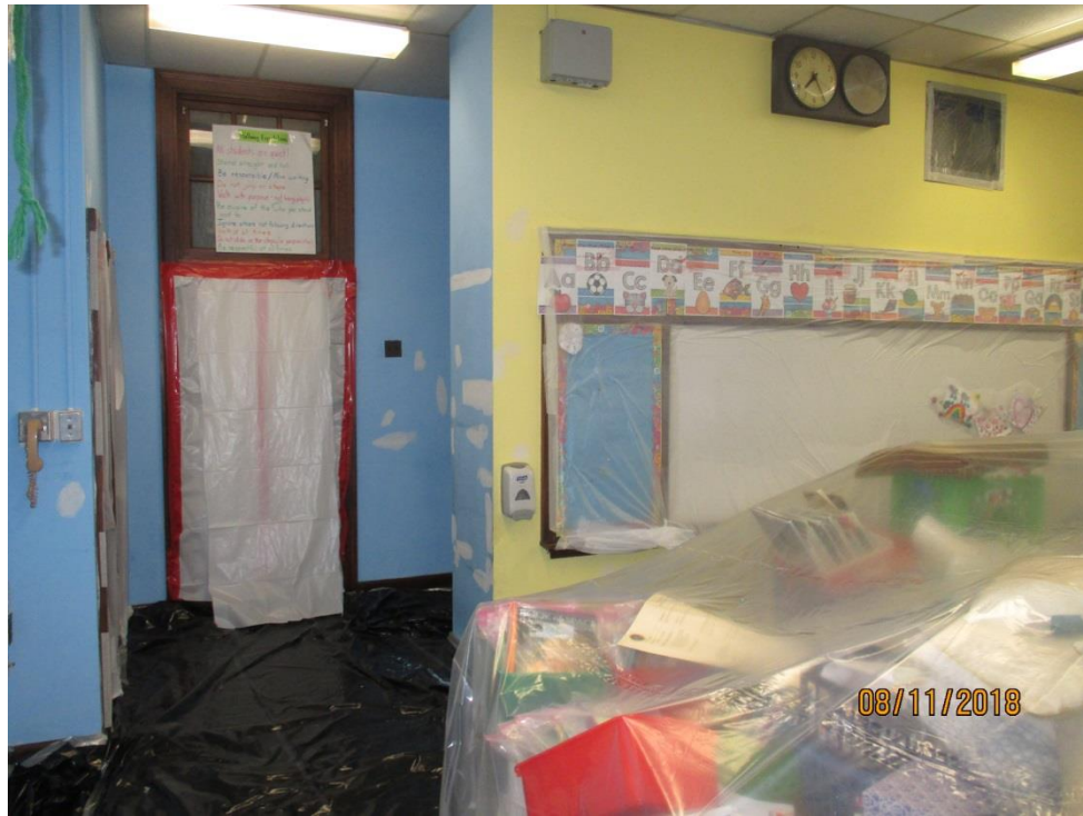
Photo 3 – Interior Containment (2-Layers): Entry Doorway to a Classroom.
