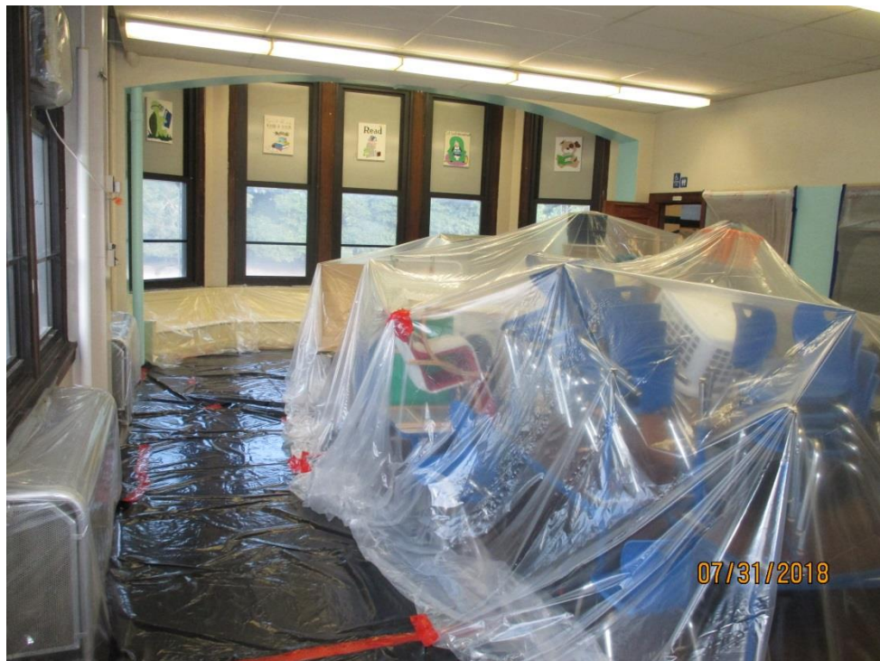
Photo 4 – Interior Containment: Cover Floors and Belongings in a Classroom.
