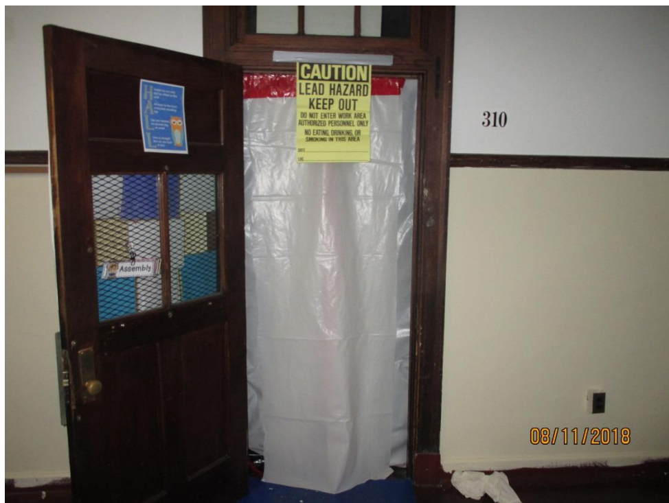
Photo 2 – Interior Containment (2-Layers): Entry Doorway to a Classroom.
