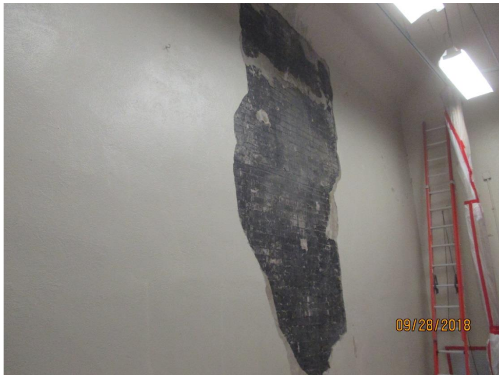
Photo 18 – Stage Wall following Scraping and Prior to Plastering/Painting.
