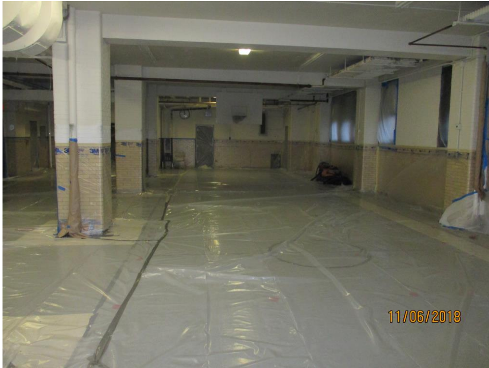
Photo 9 – Interior Containment: Cover Floors and Walls (in Gymnasium).
