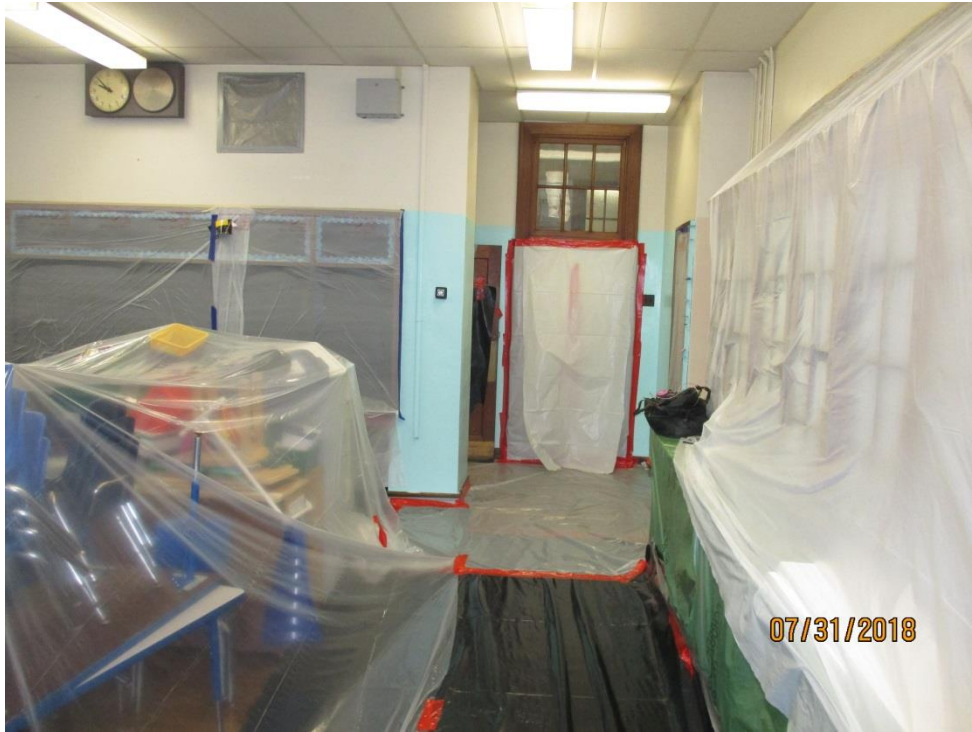
Photo 5 – Interior Containment: Cover Floors, Walls, and Belongings in a Classroom (and entry doorway).
