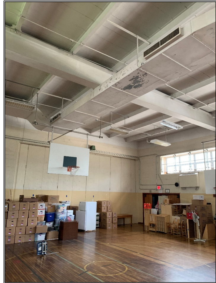
Photo 2 Lead Based Paint on Steel Beams in Gym
