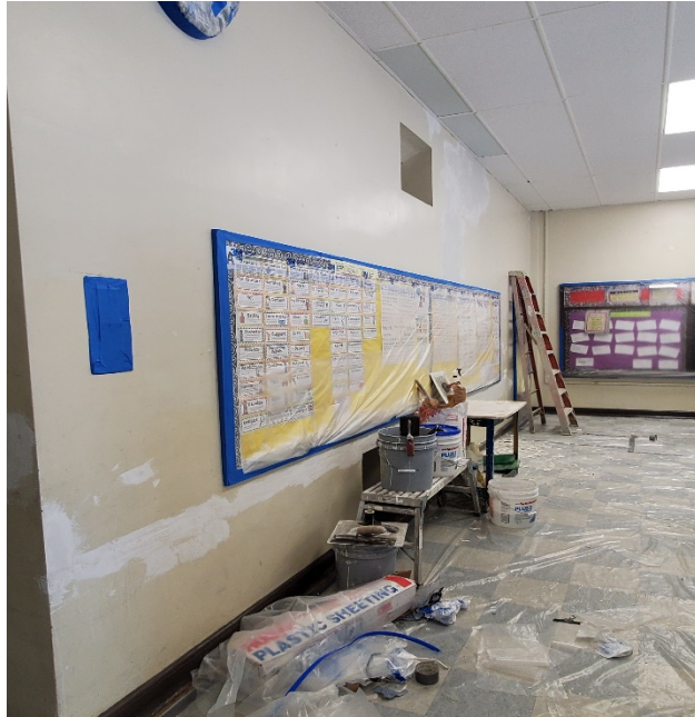
Photograph 3 – Classroom undergoing stabilization (plastering)
