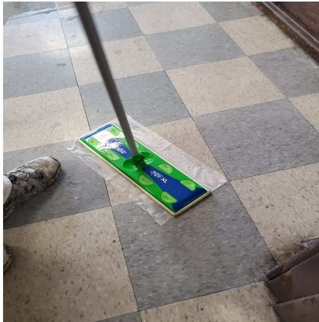
Photograph 6 – RRP wipe on tile floor
