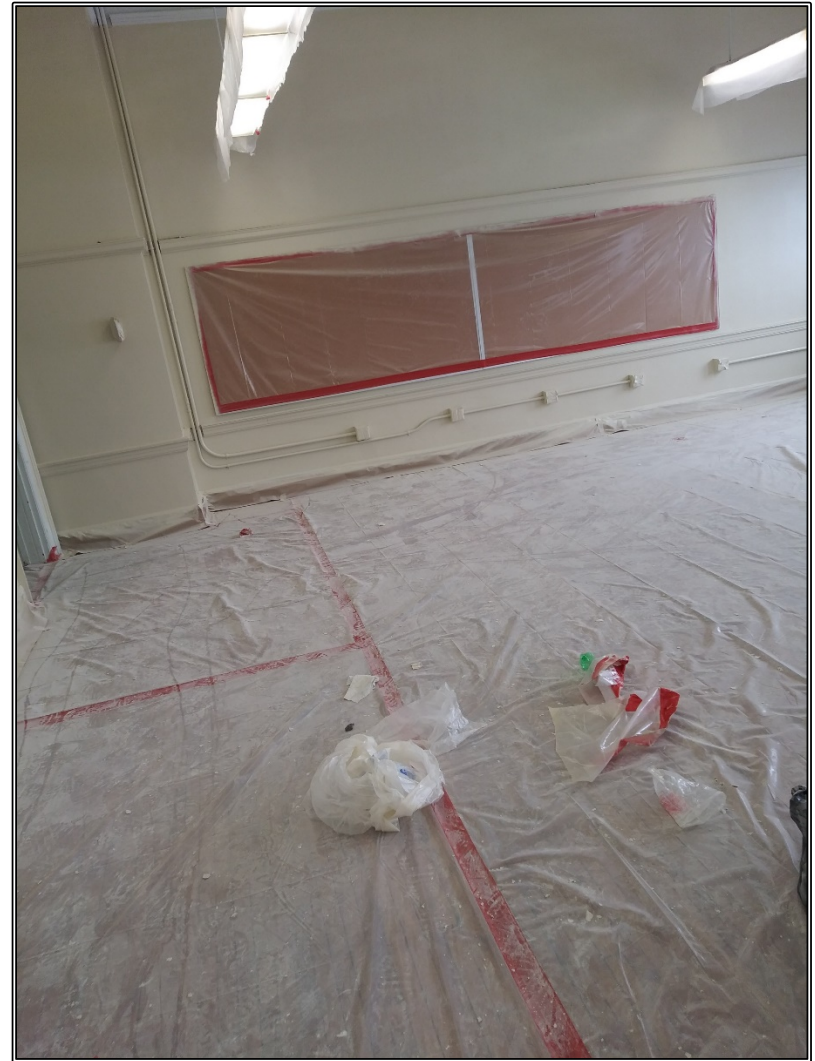
Photos 3 & 4 Typical Contained Classroom During Renovation
