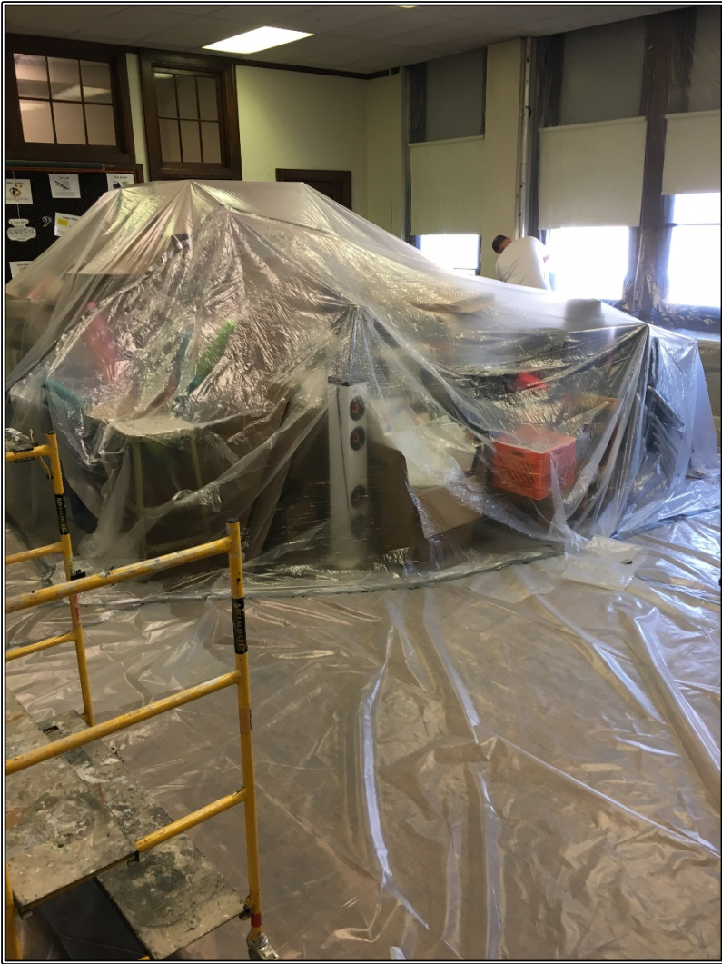
Photos 3 & 4 Typical Contained Classroom During Renovation
