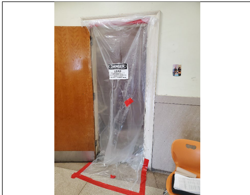
Photograph 1 – Service Closet Prep
