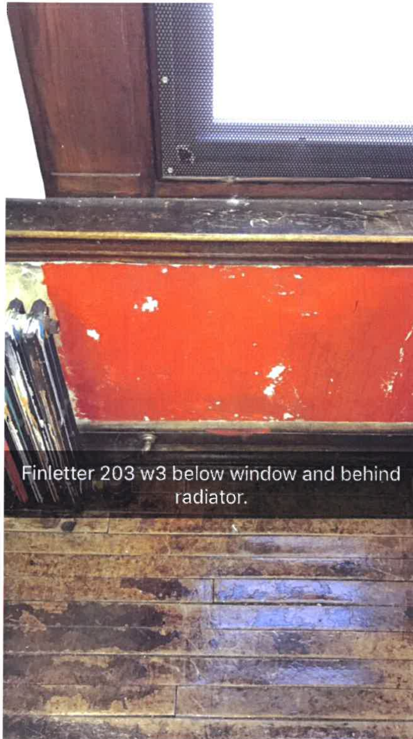
Prior to stabilization.
