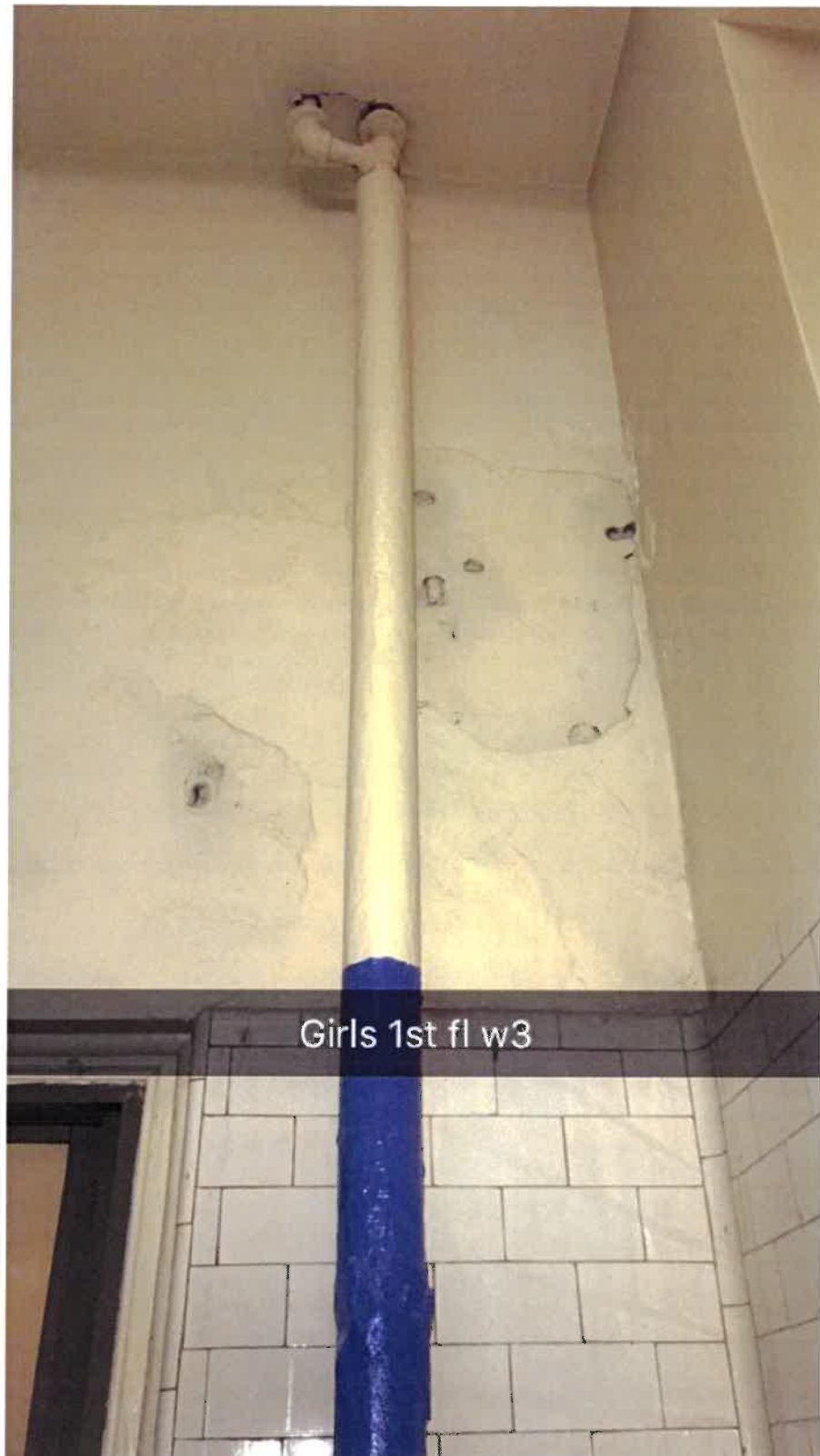
Prior to stabilization.
