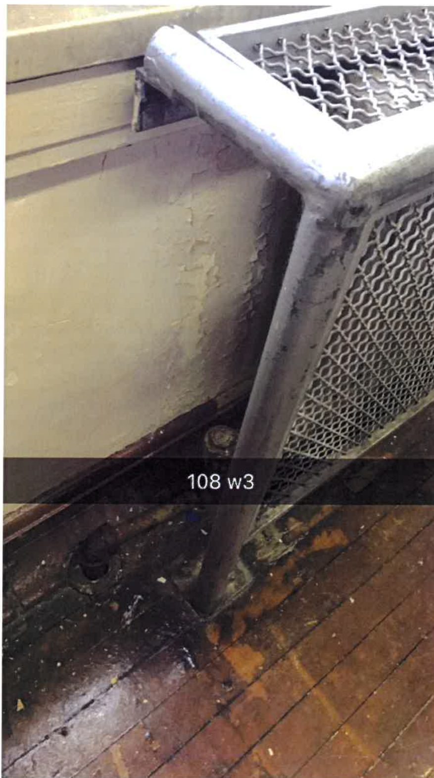
Prior to stabilization.
