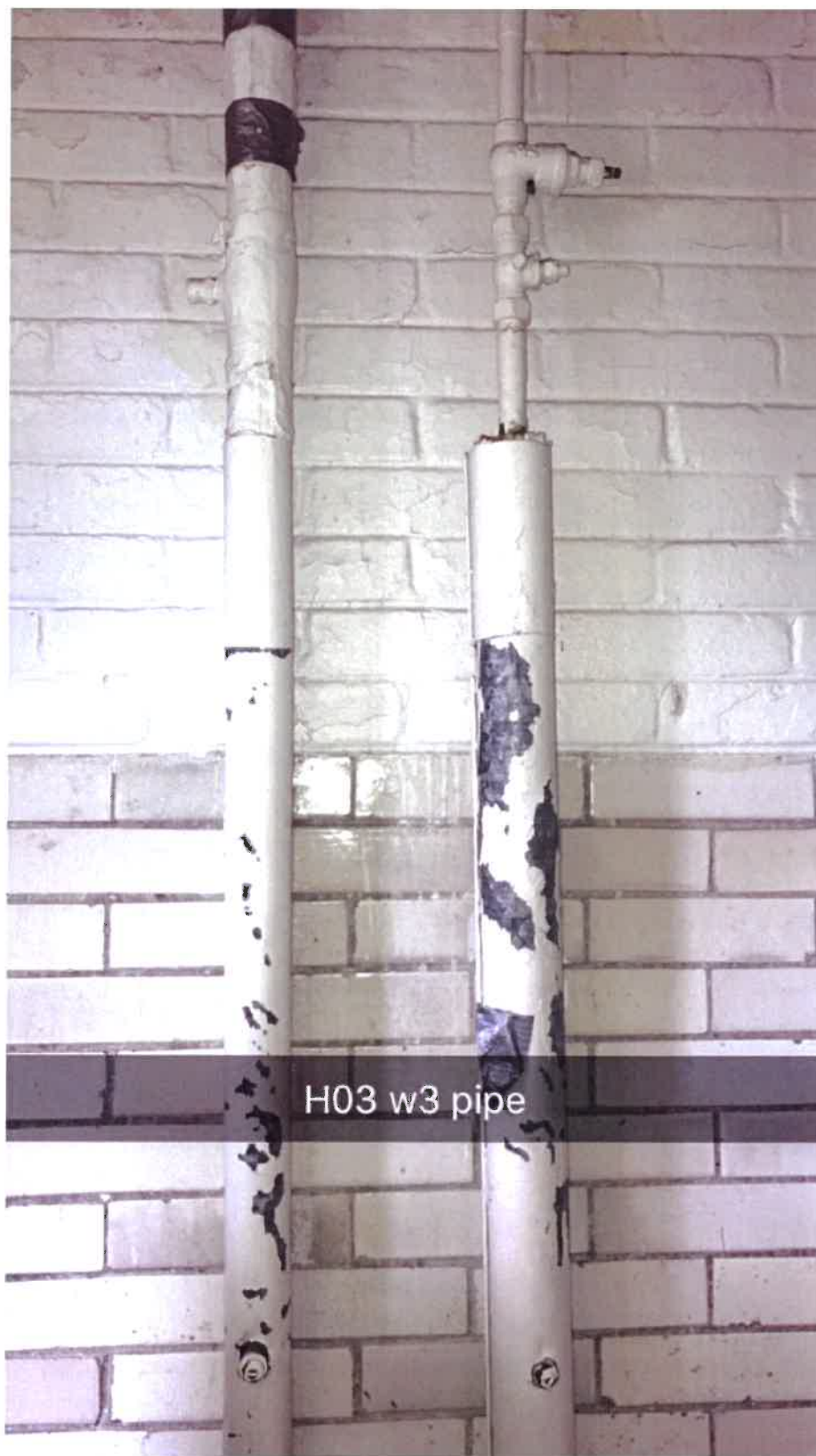
Prior to stabilization.
