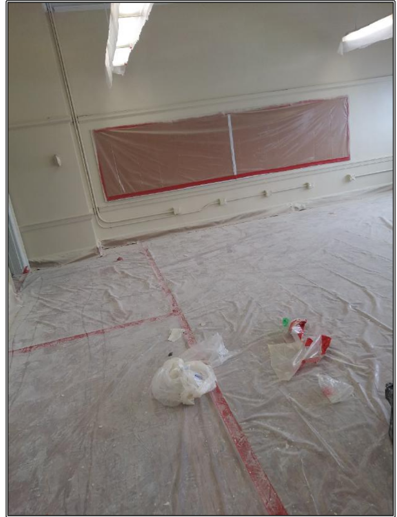
Photos 3 & 4 Typical Contained Classroom During Renovation
