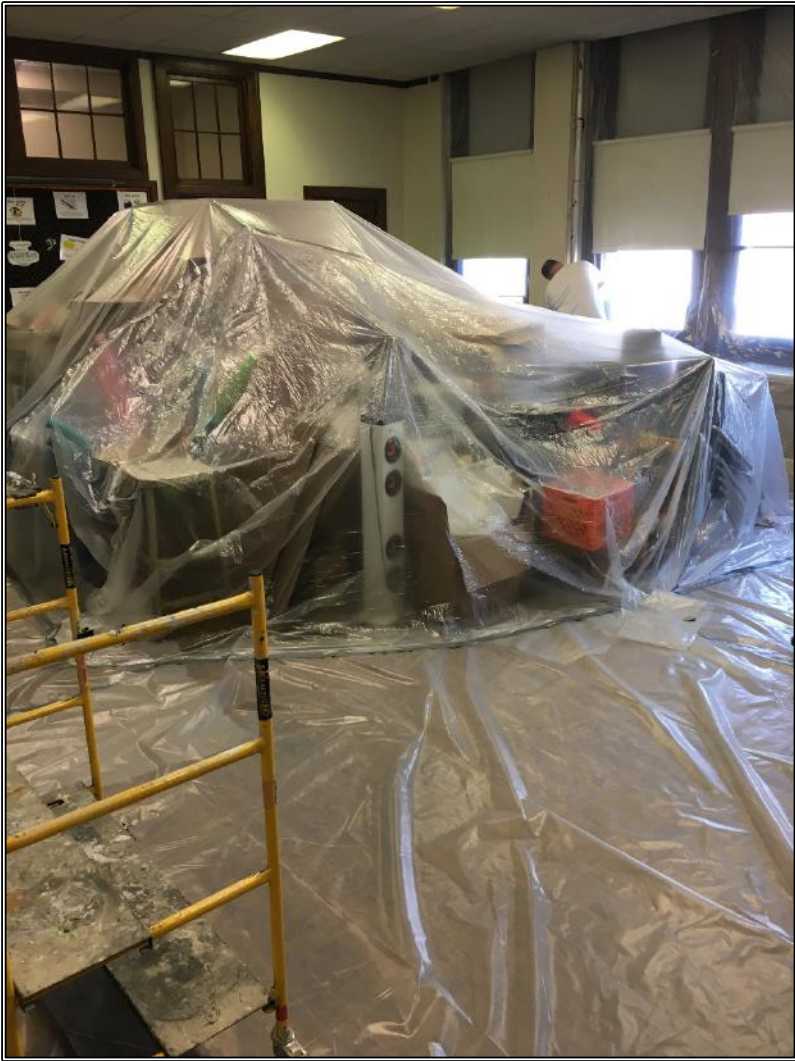
Photos 3 & 4 Typical Contained Classroom During Renovation
