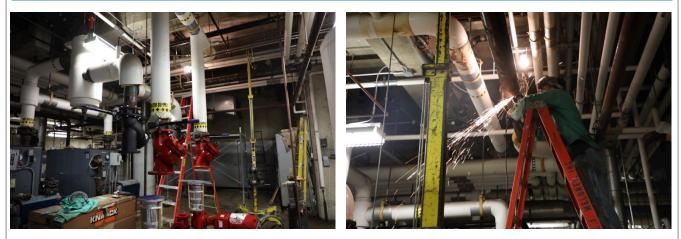
Contractors at the Munoz-Marin school are replacing over 40 unit ventilators and 11 air handlers to prevent moisture buildup that can cause mold. They are also replacing ducts to improve air quality throughout the school.
