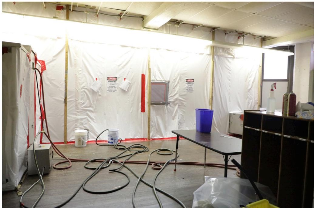
In partnership with the Philadelphia Health Department, the District sealed off a room at Olney Elementary School that was found to contain asbestos and is using vacuums with special HEPA filters to remove asbestos from the air.
