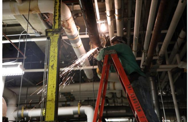
Contractors at the Munoz-Marin school are replacing over 40 unit ventilators and 11 air handlers to prevent moisture buildup that can cause mold. They are also replacing ducts to improve air quality throughout the school.
