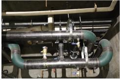
Teams at the JB Kelly school are hard at work on significant upgrades to the building HVAC system. Contractors have replaced over 2,000 linear feet of water mains and are preparing 83 unit ventilators and 7 air handlers for installation. This work will improve air quality throughout the school and prevent moisture buildup that can cause mold.
